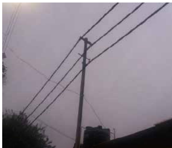
Fig 2. 3 Feeders on 1 Pole using ABC
