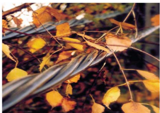
Fig. 5. ABC Cable Passing Thru Trees (Courtesy – Ensto India Pvt. Ltd.)
