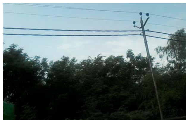
Fig 3. 2 ABC Feeders + 1 ACSR Feeder
