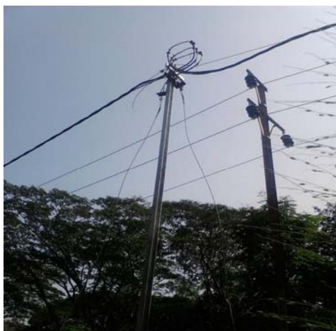
Fig 1. Mid Span Joint in ABC Feeder
