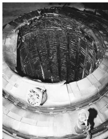
Figure 1 – Damage to inside of coil winding stack of oil-filled transformer
