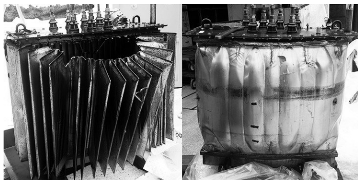
Figure 3 – Transformer tank fault
