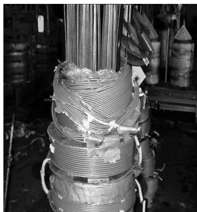
Figure 2 – Transformer interturn fault
