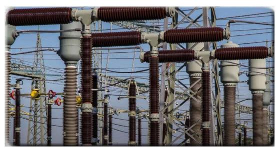
All outdoor switchyards for HV, EHV, comprised of AIS substation. An air-insulated substation (AIS) is one where the main circuit potential is insulated from the ground by air using porcelain or composite insulators and/or bushings.
