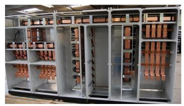
**Function:** Conduct electricity within the substation.
