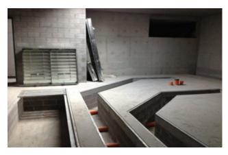
Cable trenches and raceways are essential for organizing, protecting, and routing electrical cables within an indoor substation.
