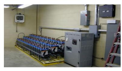
**Purpose:** Provide backup DC power for control, protection, and communication systems.
